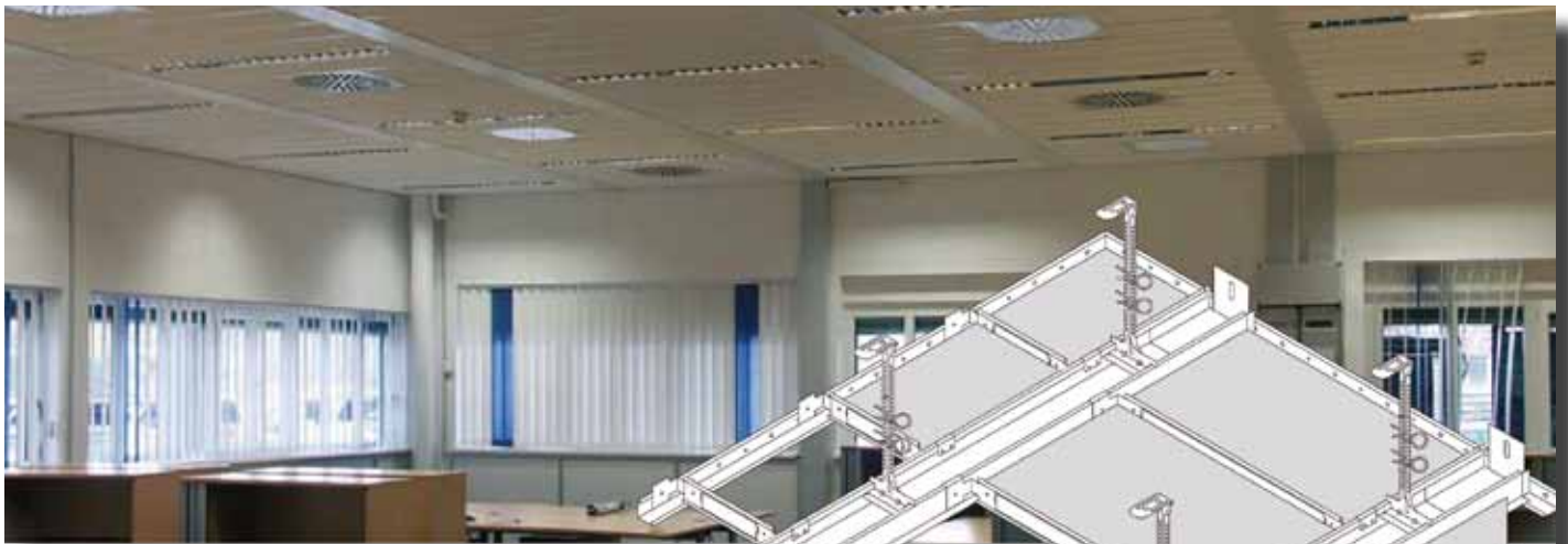
Meeting required tolerances guarantees a comfortable fit between the different sections and materials used in suspended ceiling structures.
